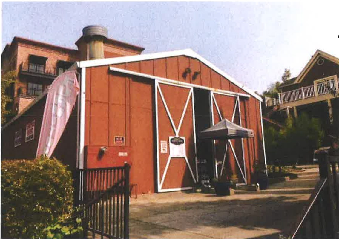
FIGURE 4: COMMERCIAL BUILDING AT 608 ½ SUTTER STREET
